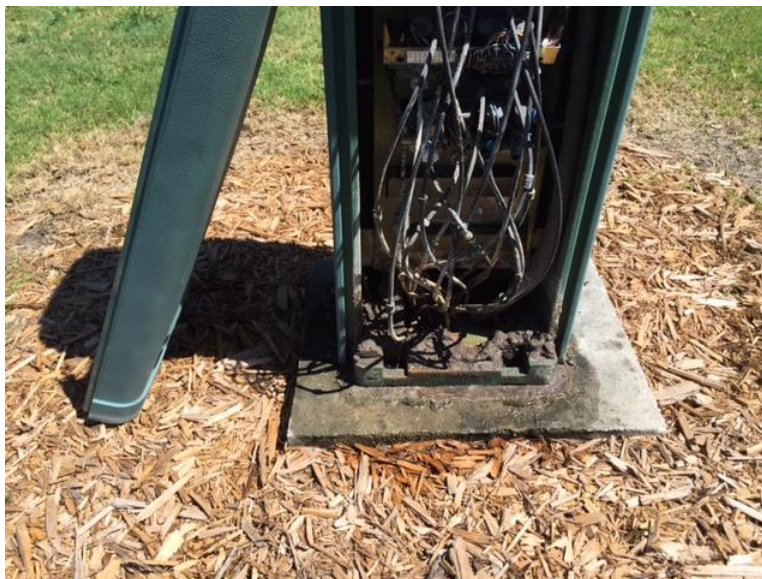
Irrigation controllers have some hydraulic issues of leaking which can lead to heads running all night or pressure issues if not addressed
